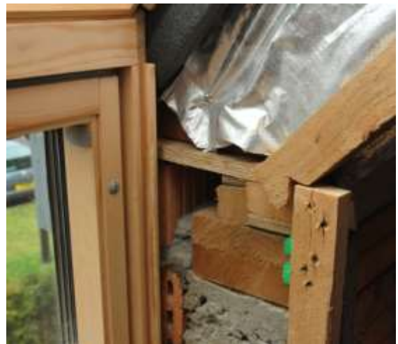
Fig. 3. Real details – typical roof/wall junction.
