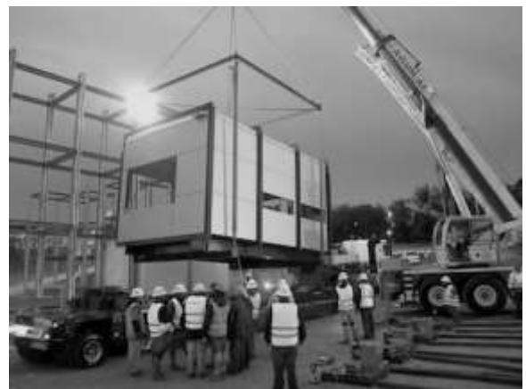
Fig. 4. Lifting and placing the living room module (photograph by Clay Anderson)
