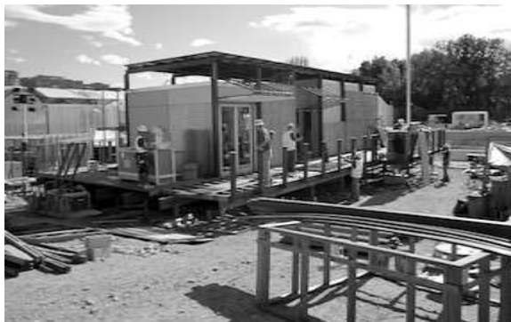
Fig. 2. Construction well underway on the competition site (photographs by Clay Anderson)
