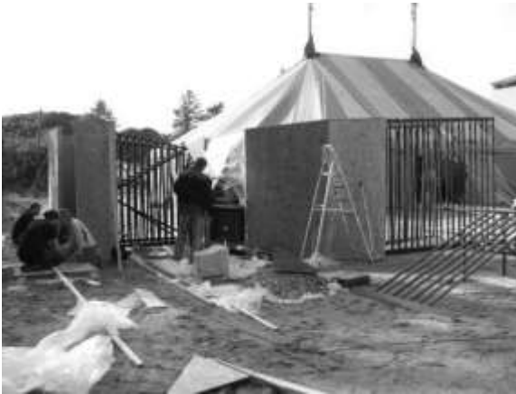
Fig. 1. Kraftka under construction
