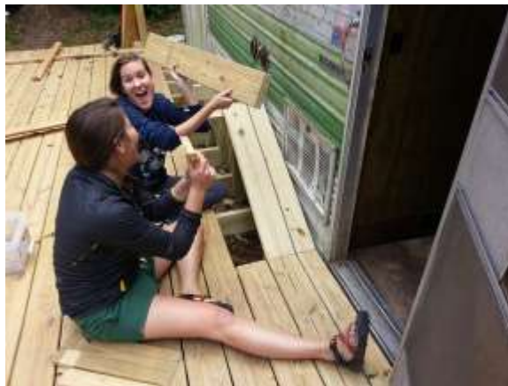
Fig.4. Students assembling the deck's folded bench (photograph by author)
