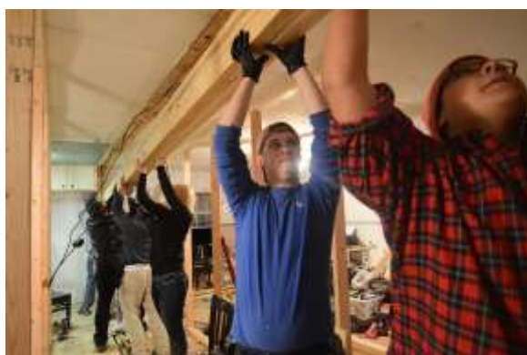
Fig. 2. Renovation of mobile home interior: (top) temporary framing between living spaces, (bottom) installation of central beam to open the living area (photograph by Alex Sanchez)
