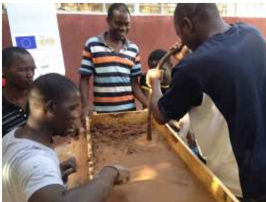
Fig. 2. Completing the first poured earth wall
