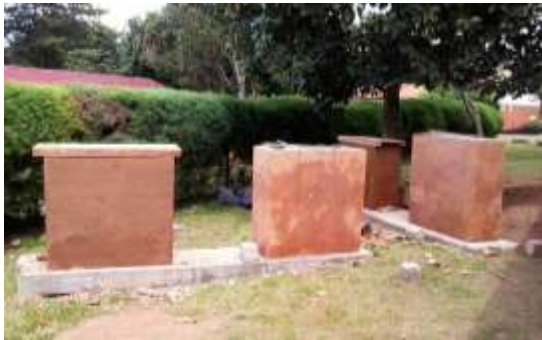
Fig. 3. The completed poured earth walls
